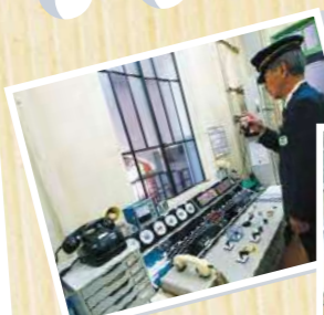
The hoist controls in the operator's room at Cable Enryakuji Station
